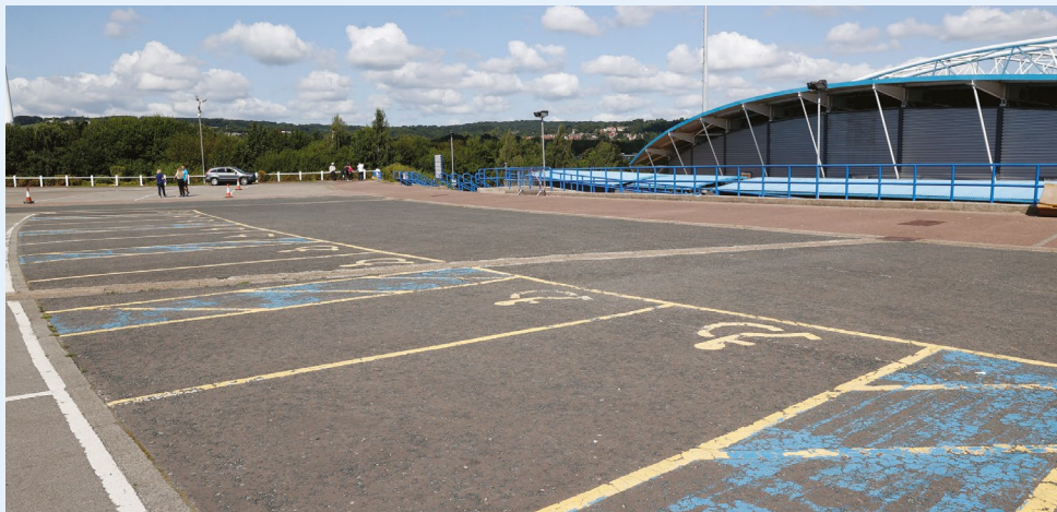
Figure 4 Disabled car parking spaces in the St Andrew's Road car park upper level adjacent to the Magic Rock Stand
