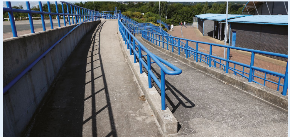
Figure 5 Ramp leading from St Andrew's Upper Level car park to the Magic Rock Stand
