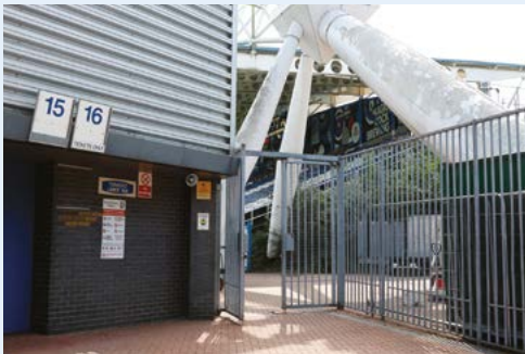
Figure 18 Accessible Entrance next to Turnstile 16
