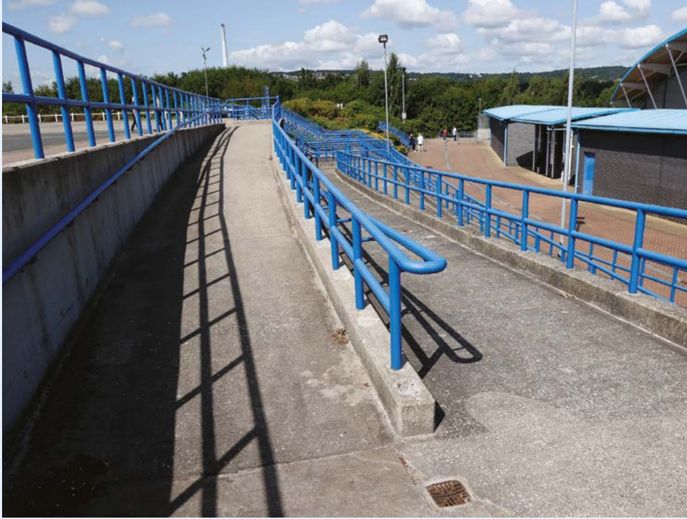
Figure 17 Ramp leading from St Andrew's Upper Level car park to the Magic Rock Stand
