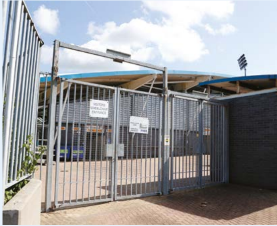
Figure 20 Accessible entrance next to turnstile 17
