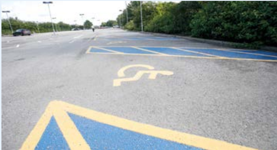
Figure 2 Town Avenue car park disabled parking bays
