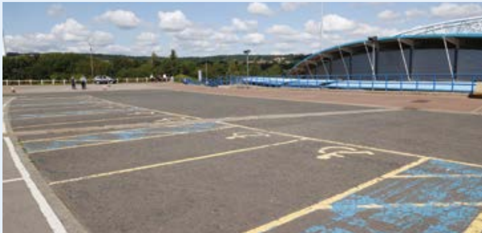
Figure 4 Disabled car parking spaces in the St Andrew's Road car park upper level adjacent to the Magic Rock Stand
